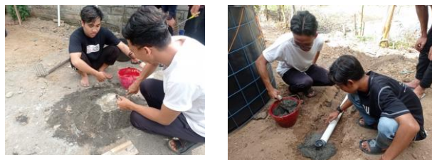
Picture 5. Installation of Water Outlet
