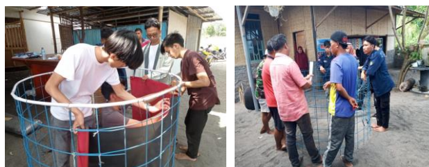
Picture 3. Installation of Tarpaulin Pond Frame
