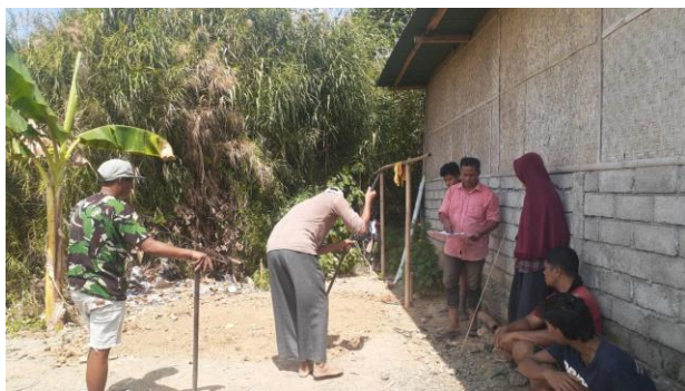
Picture 1. Land Preparation for Tarpaulin Pond
