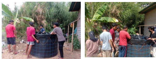
Picture 4. Placement of Tarpaulin Pond on The Land
