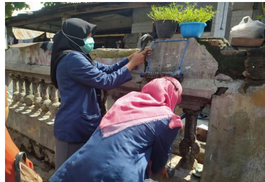
Gambar 3. Instalasi wadah tanam
