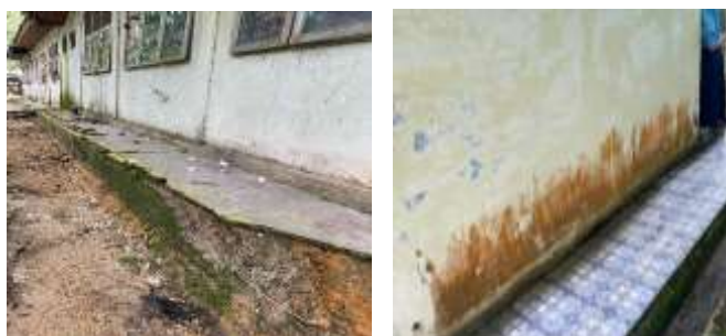
Figure 4. (a) The land is sinking, (b) Peeling wall paint
