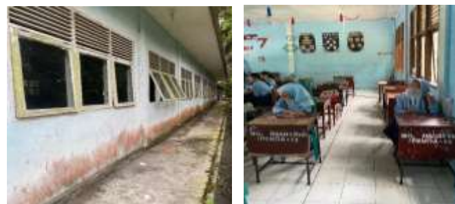
Figure 5. (a) Windows that can't be closed, (b) The classroom floor is sloping
