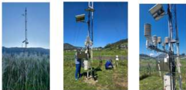
Figure 3. Field view of the Automatic Weather Station (AWS) on the Dieng Plateau, Central Java
