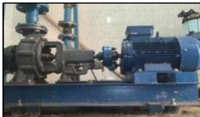
Figure 5. Horizontal end suction centrifugal pump 2-3 l/d
