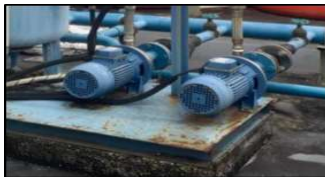
Figure 6. Horizontal end suction centrifugal pump 2-3 l/d
