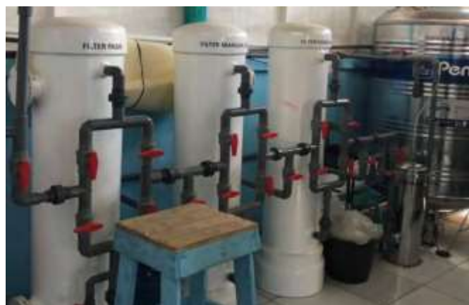
Figure 3. Filtration process (sand filter, manganese zeolite filter, activated carbon filter, and cartridge filter)
