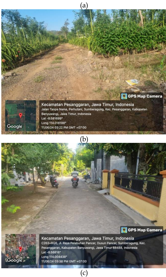
Figure 7. Types and Conditions of Roads Around Pancer Banyuwangi (a) Cast Road (b) Solid Land Road (c) Paving Block Road
